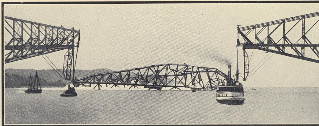
The collapse of the suspended span at 10.50 a.m. on the 11th September, 1916
