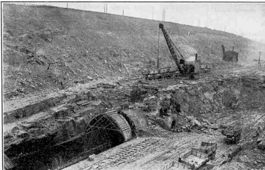
The Solid Sandstone through which Chevet Tunnel ran
