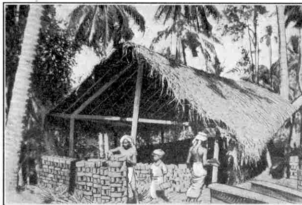
Fig. 2. Stacking the Bricks
