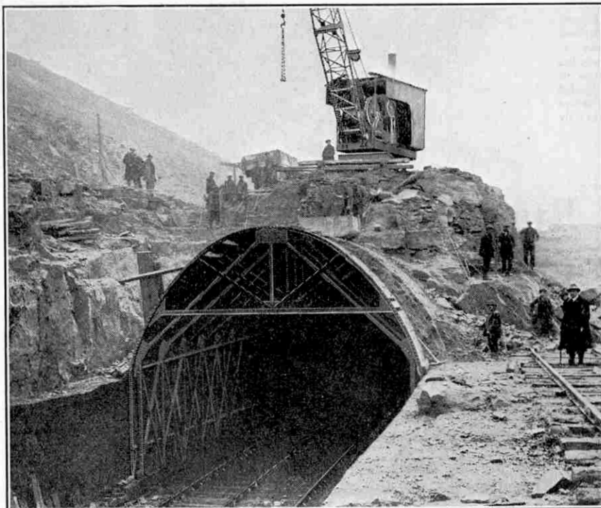
The operations at Chevet Tunnel in progress
