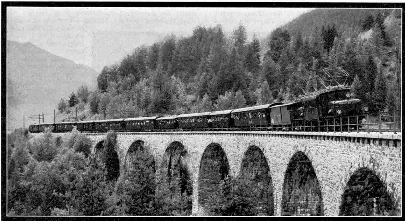
1000 h.p. Electric Loco hauling 200 ton train over the mountain stretch between Tiefencastel and Filisur
