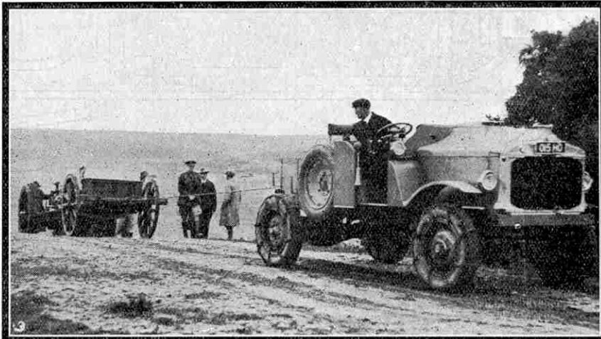
The "Hathi" hauling a heavy howitzer up a hill in recent War Office tests
