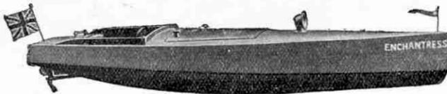
(Runs 4 hours on a 6d. lamp battery). The hull is built of specially selected mahogany, 25" long, enamelled white above the water line and green below. The boat is fitted with a powerful self-starting motor, operated by a miniature turnbuckle switch in the cabin and a brass double-blade propeller threaded on the shaft. Price 31/6. Batteries 6d. each.
