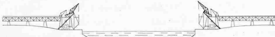
The first panel of the arch being erected by 120-ton creeper cranes. Note the first anchorages from the top of the end posts. (Further progress will be illustrated in future issues)
