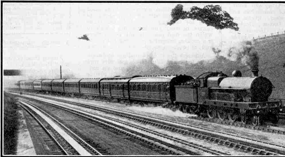
Third part of L.M.S. 10 a.m. Scotch Express (4-6-0 Loco No. 2427) at Bushey
