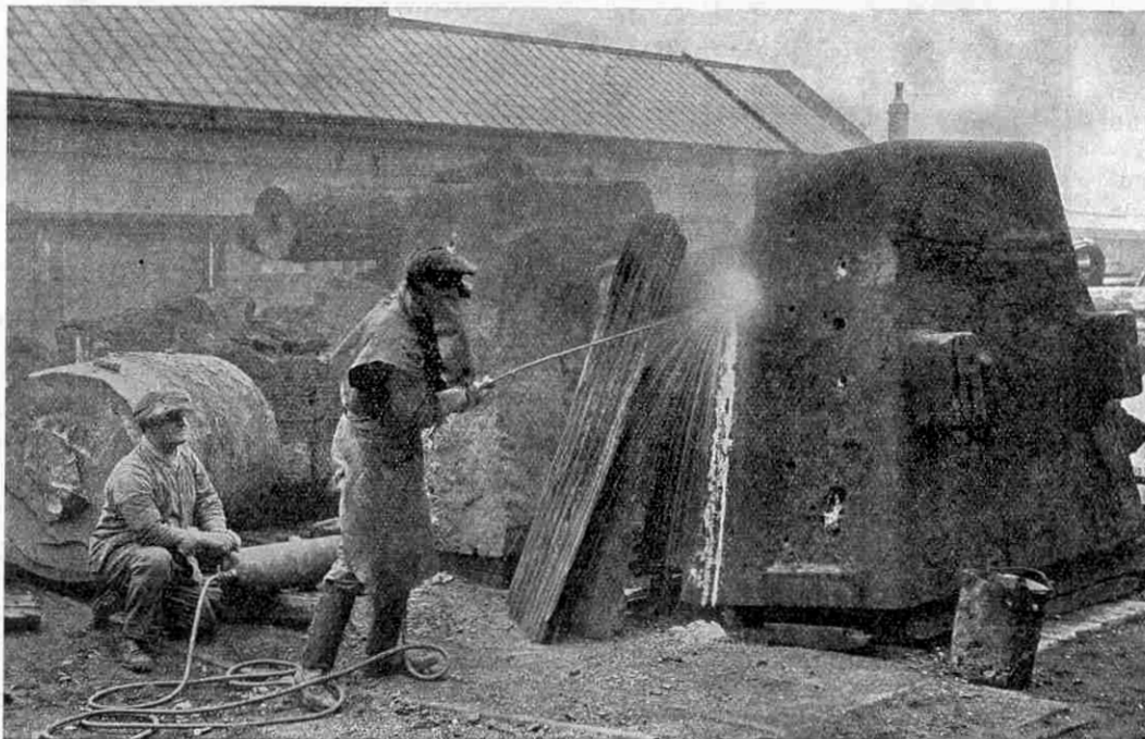
Boring holes with a jet of oxygen in a solid steel casting in readiness for breaking it up by exploding charges of dynamite within it
