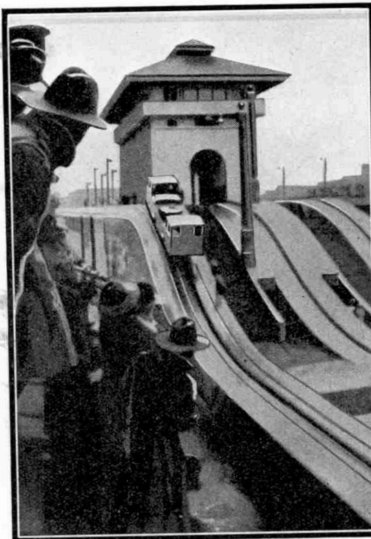
The electric mule descending one of the ramps on the Pedro Miguel Lock. The building in the rear is the control house
