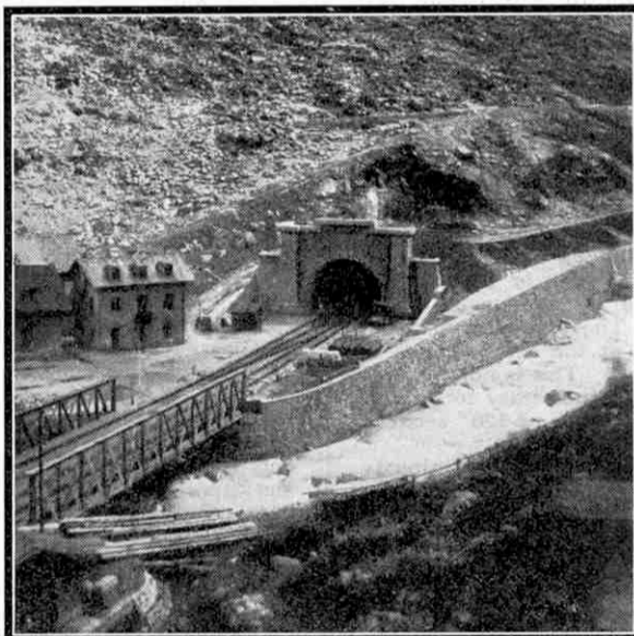
The Northern Portal of the St. Gotthard Tunnel
