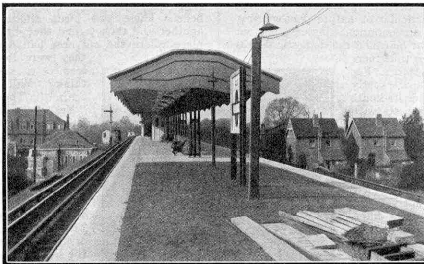
A good design for an Island Platform Station
