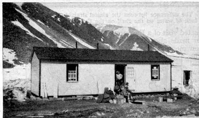
The Royal Canadian Mounted Police Post at Craig Harbour, Ellesmere Land, after being newly painted by the men (see above)
