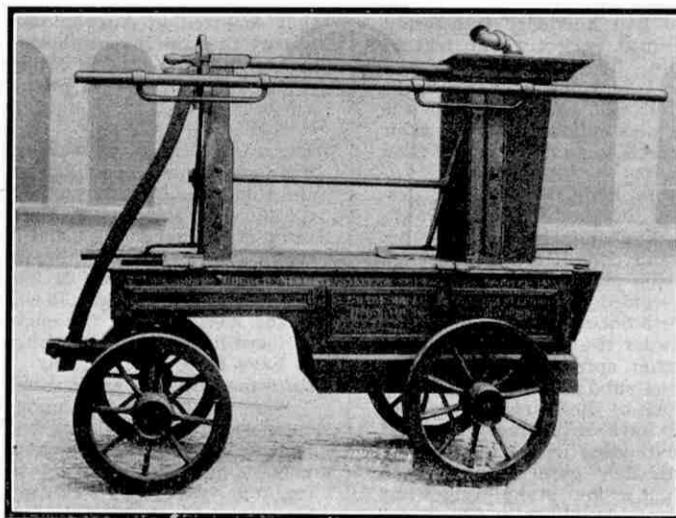
A good example of the early hand-pump fire engines
