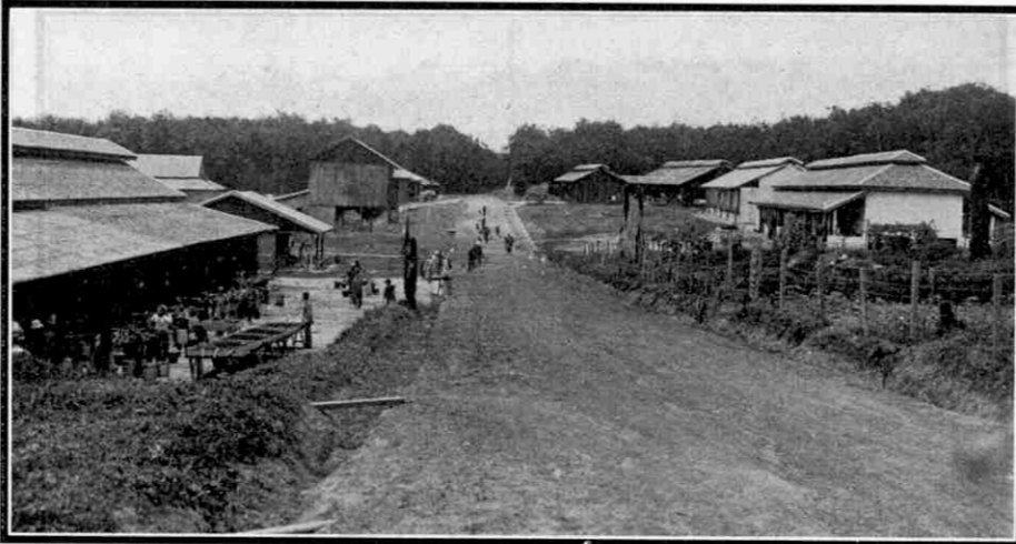
General view of the central building site at a plantation. Note the coolies delivering latex at the factory on the left
