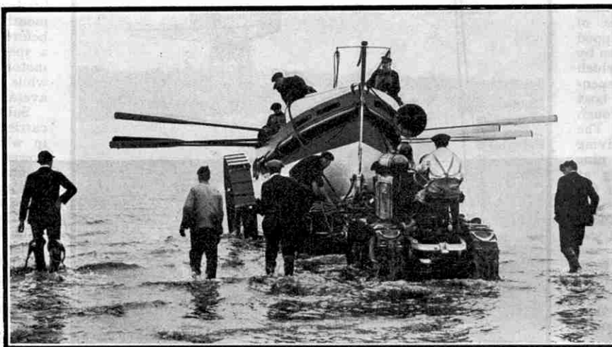
Another view of a launch showing the tractor actually in the water
