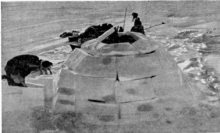
Placing the last block but one in position. From the "Book of Polar Exploration" reviewed on this page.
