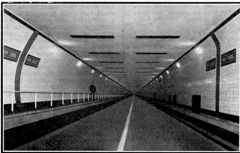
The halfway line! The vertical lines of coloured tiles mark the boundary between the states of New York and New Jersey. This portion of the tunnel is about 16 ft. below the bed of the Hudson River.
