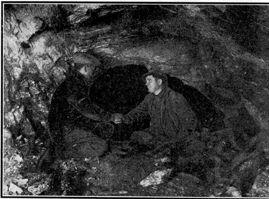
Underground greetings! Tunnel workers shaking hands after "holing through" when the sections bored from opposite sides of the river met.
