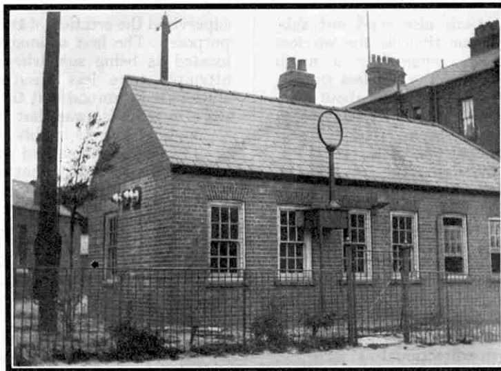
A Coast Station with a directional receiving aerial of the small single loop pattern.
