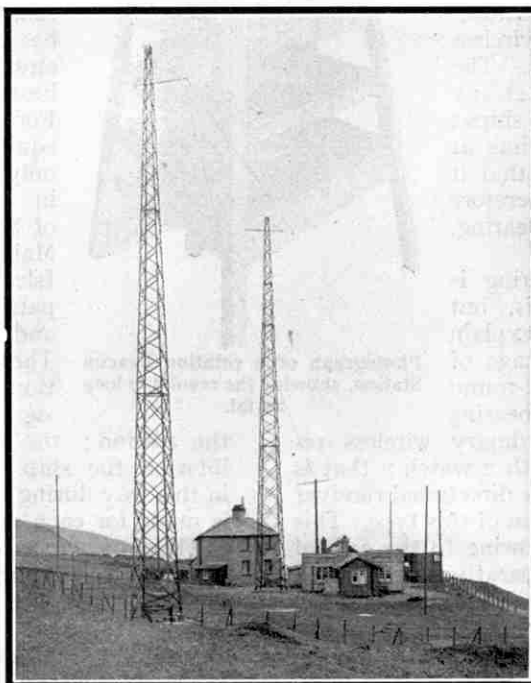
View of another Coast Station showing the short masts that stay out a directional receiving aerial of the large double loop pattern.
