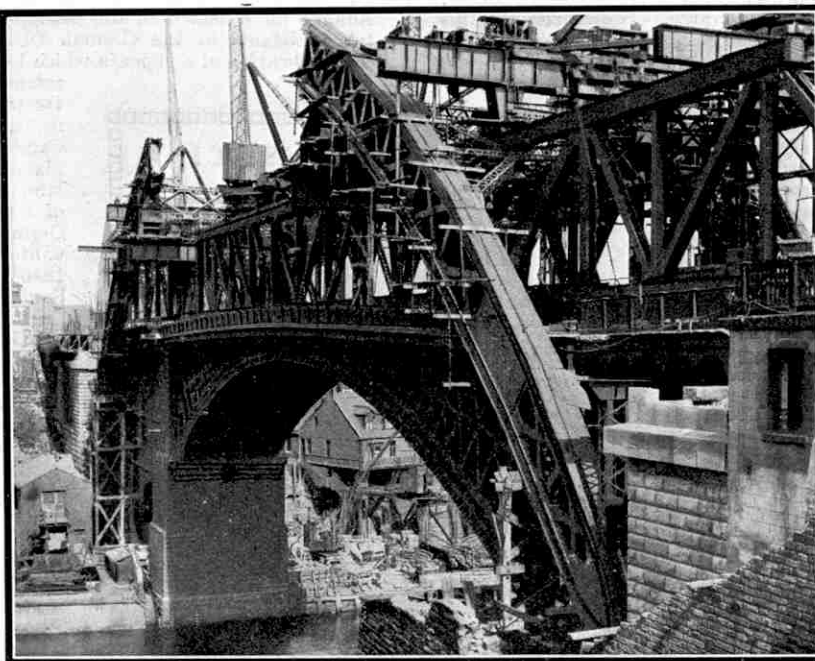
The building of Wearmouth Bridge; the arch ribs in course of erection. For this and the other photographs illustrating this article we are indebted to the courtesy of Sir William Arrol and Co. Ltd.
