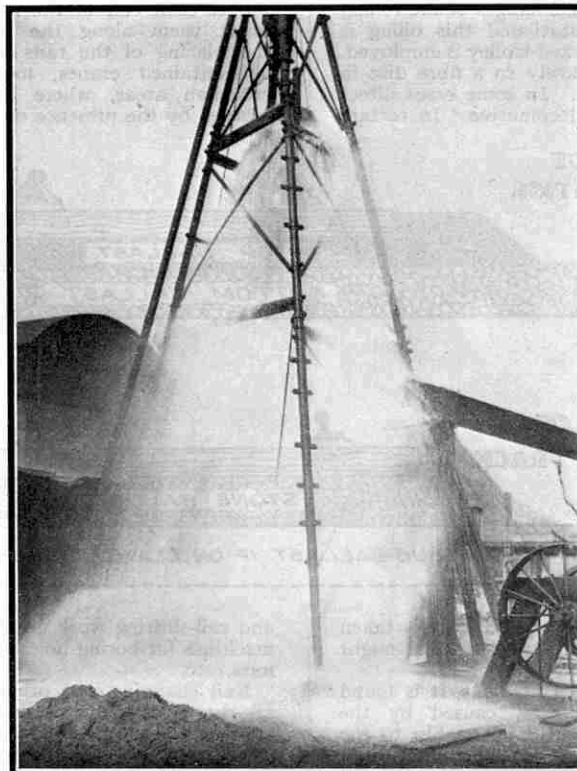
Courtesy [C. Isler & Co. Ltd.] A column of water 30 ft. in height that escaped from an artesian well recently bored at Slough. The overflow of 250,000 gallons per hour is believed to be the largest ever obtained from a well in this country.
