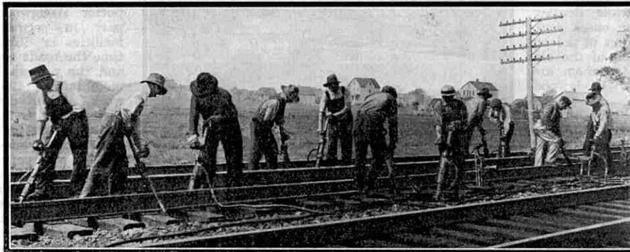
Ballast tamping with 12-unit compressed air machine.
