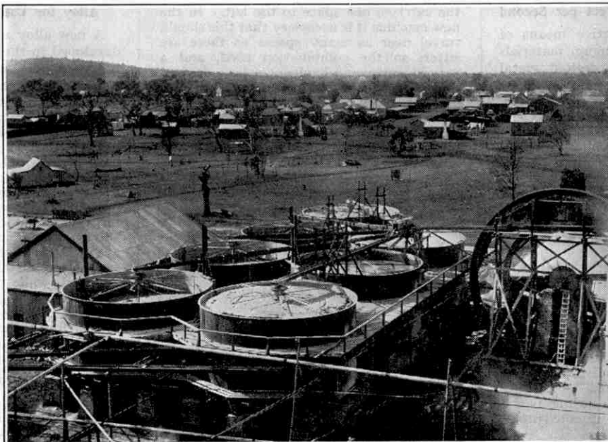
A typical scene at an Australian gold mine, showing the tanks in which potassium cyanide solution extracts gold from the crushed ore.
