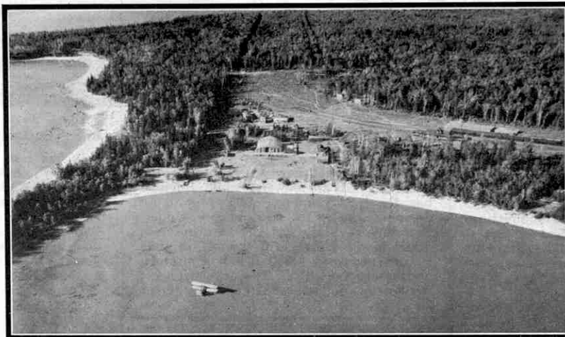
The air station at Victoria Beach, Manitoba.
