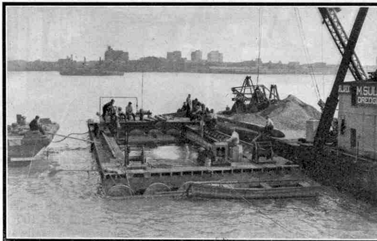
The grill for smoothing the sand bed. The sand and the lowering buckets are shown on the right.
