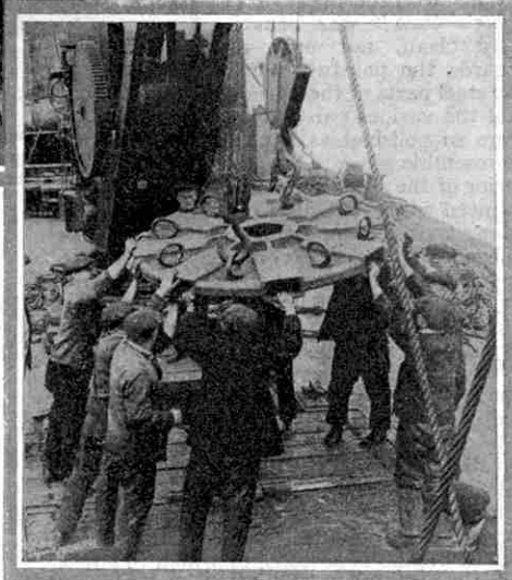
(Top) Screwing operations in progress. The giant capstan being turned by means of steam winches. (Centre) Lowering the first length of shafting, with the mooring screw chain attached, through the well of the keel. (Right) Shipping the capstan head. This is fitted on to the uppermost length of shafting, and the capstan bars are inserted in the square sockets.
