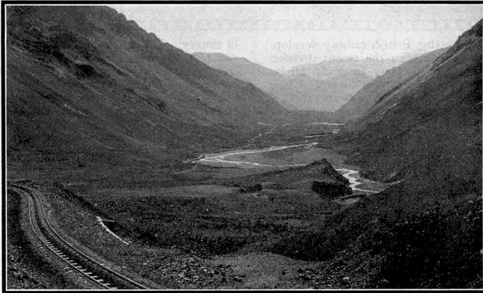
A section of the line through the Valley of the Paramillos where the gradient is so steep that it necessitates the use of the cog and rack system.
