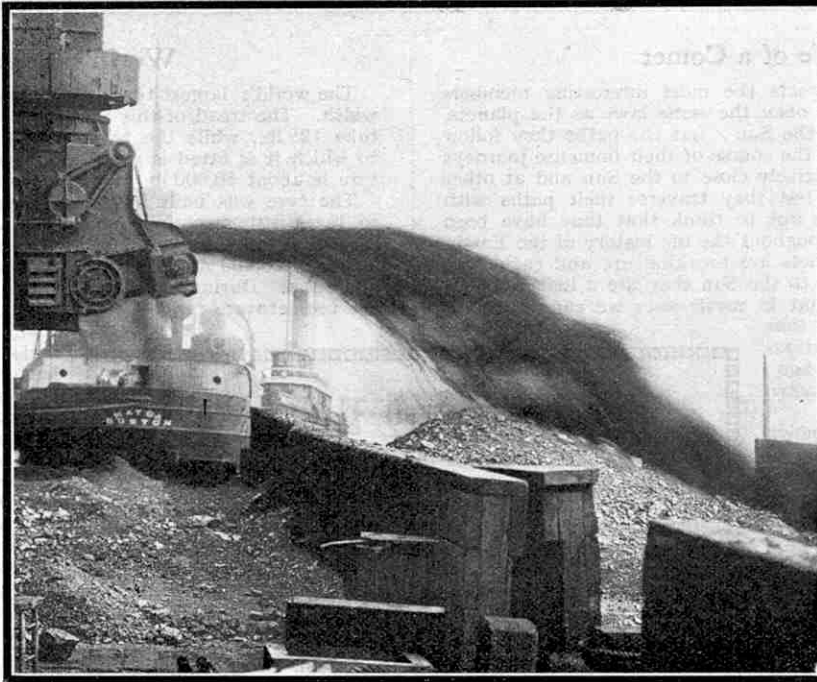
High speed coal dumper at work at the Curtis Bay, Baltimore, pier of the Baltimore and Ohio Railroad. The plant is one of the largest of its type in the world, and has a capacity of 4,000 tons per working hour, or 10,000 tons per year under normal conditions. It was described in the "M.M." for March 1929.
