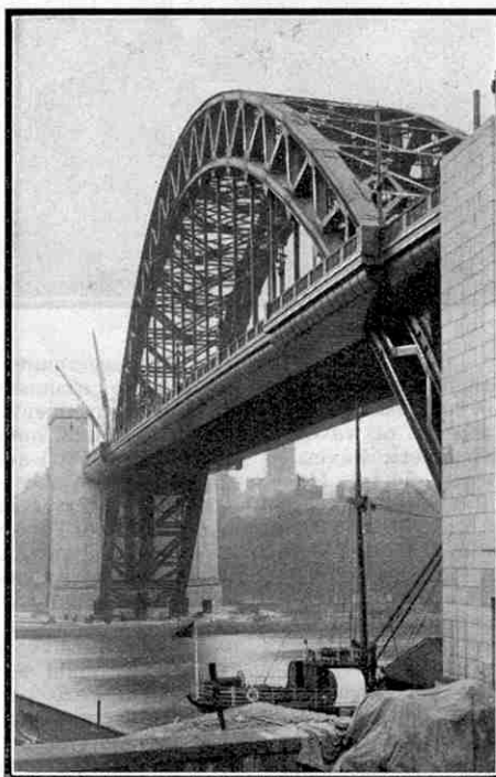
Another view of the bridge. The crown of the arch is 170 ft. above the level of the river, and the deck allows a clear height for shipping of 84 ft. 6 in.
