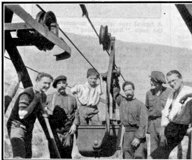
The head of the aerial ropeway down which iron ore is carried from the mines at Escoums, in the Pyrenees.
