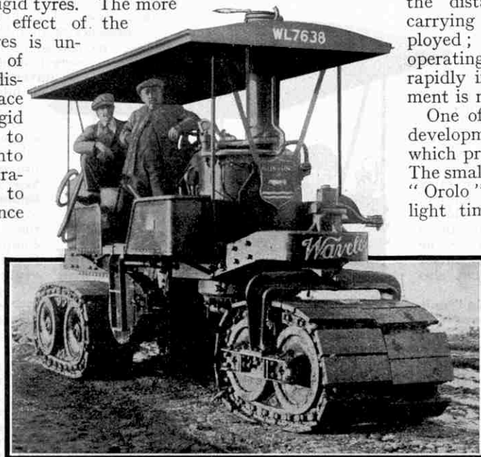
"Waveless" roller fitted with girder track, which consolidates the surface without producing "waves."
