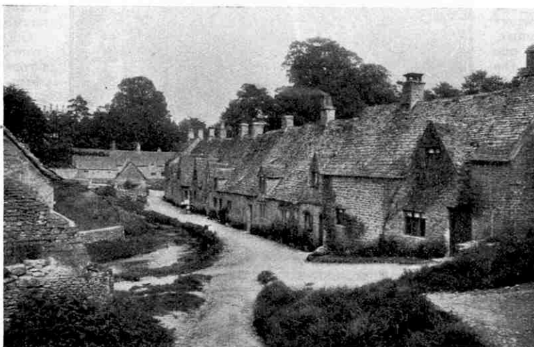
Arlington Row, Bibury, showing limestone slabs often used for the roofs of cottages in the Cotswolds. (From "Rediscovering England" reviewed on this page).
