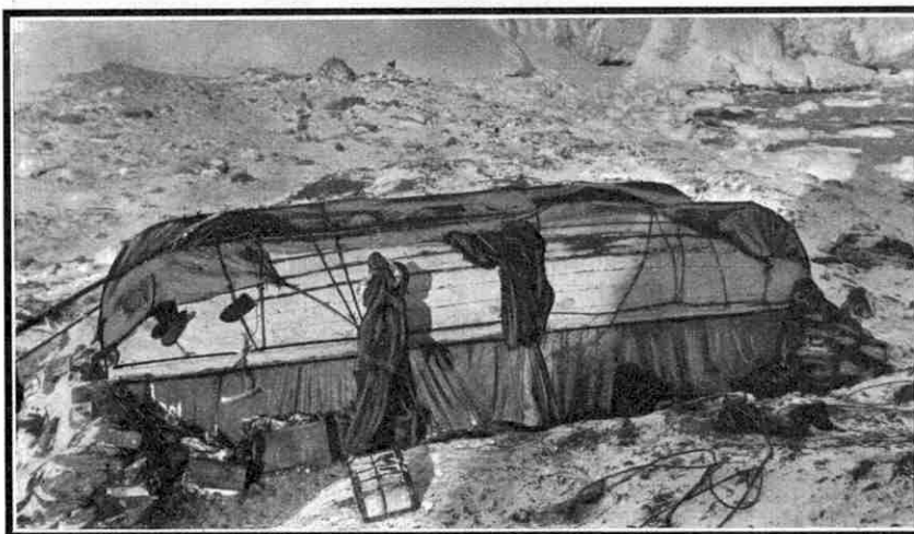
The hut on Elephant Island in which the crew of the "Endurance" lived for four months. It was made by placing two boats upside down on walls built of rough stones.
