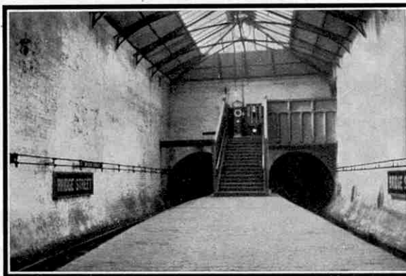
A station on the Glasgow District Subway. The conductor rails for electric lighting current may be seen on the walls. (See next page).
