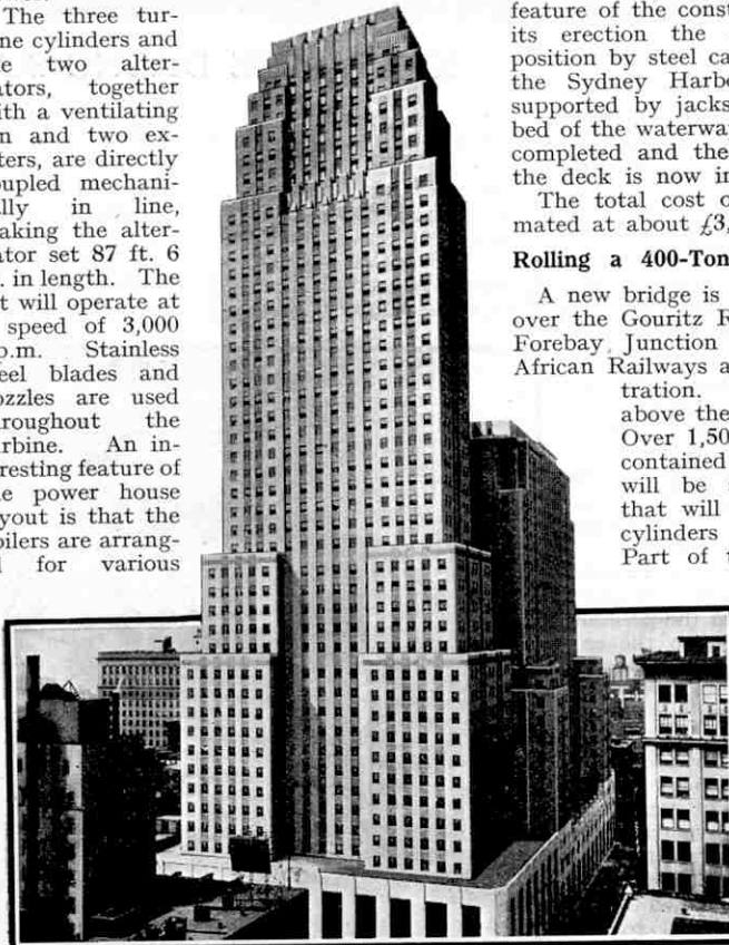
The Carew Tower, Cincinnati, Ohio. This great building is equipped with 41 elevators, six of which travel at a speed of 900 ft. per minute. Photograph by courtesy of the Westinghouse Electric Company.
