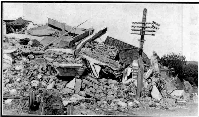
The utter ruin of the Napier Nurses' Home, a five-storey brick structure, in which many nurses were killed or injured.
