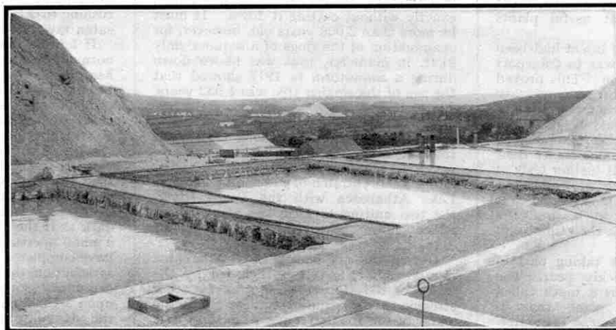
The settling ponds where, by evaporation, the clay is separated from the water, which finally runs out quite clear.
