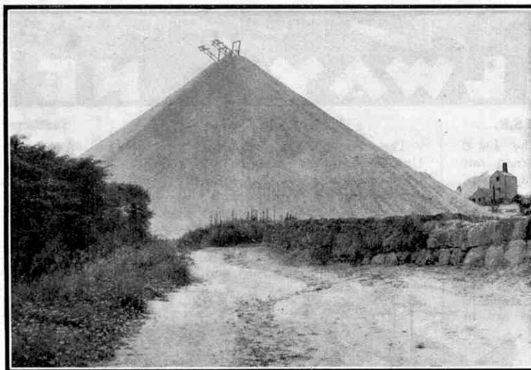
A typical 200-ft. mound of "overburden" or refuse from a china clay mine. At the summit may be seen the projecting terminus of the inclined railway up which the refuse is carried.
