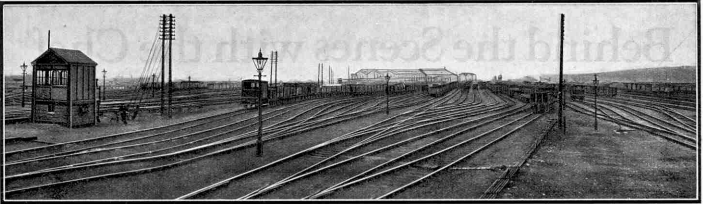
A maze of steel rails! Modern methods of steel construction have made possible huge sidings such as the one depicted here, with elaborate systems of points and crossings all working with perfect accuracy.
