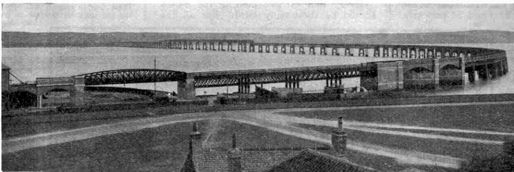
The Tay Bridge built by Sir William Arrol, whose story is told in "The Romance of Million-Making" reviewed on this page.
