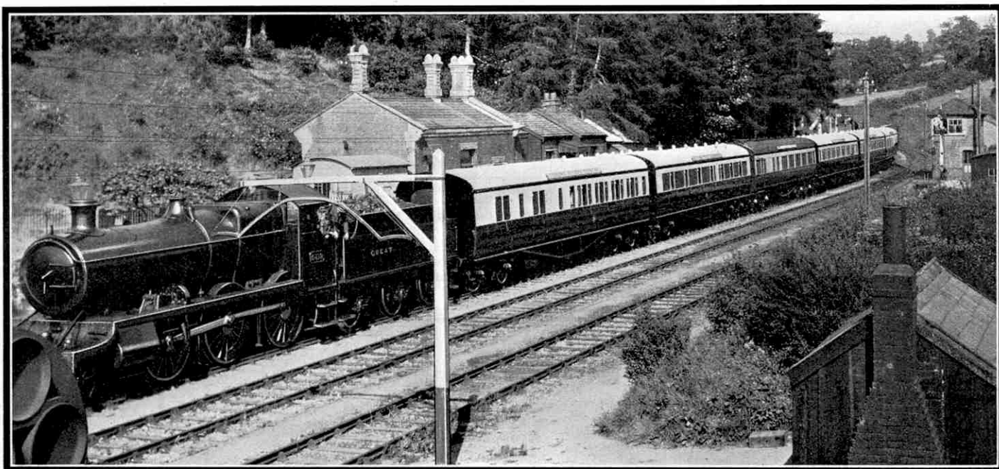
One of the locomotives and trains used when filming "The Ghost Train." This train represents the "Cornish Riviera Express" and is standing at a station on a disused branch line near Bath, where a number of scenes in the film were shot. The station was altered to represent "Fal Vale," where part of the action of the film takes place. (See page 952).
