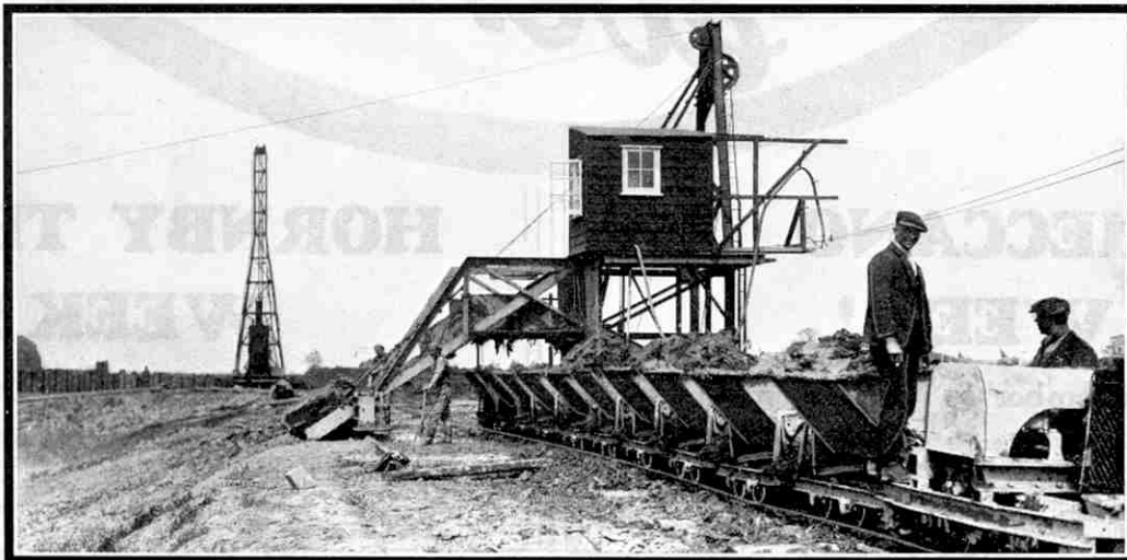
The head carriage of the Henderson Cable Drag-Scraper, with the bucket about to ascend the ramp. The tall structure in the background is a pile-driver. For this photograph we are indebted to the courtesy of John M. Henderson & Co. Ltd.
