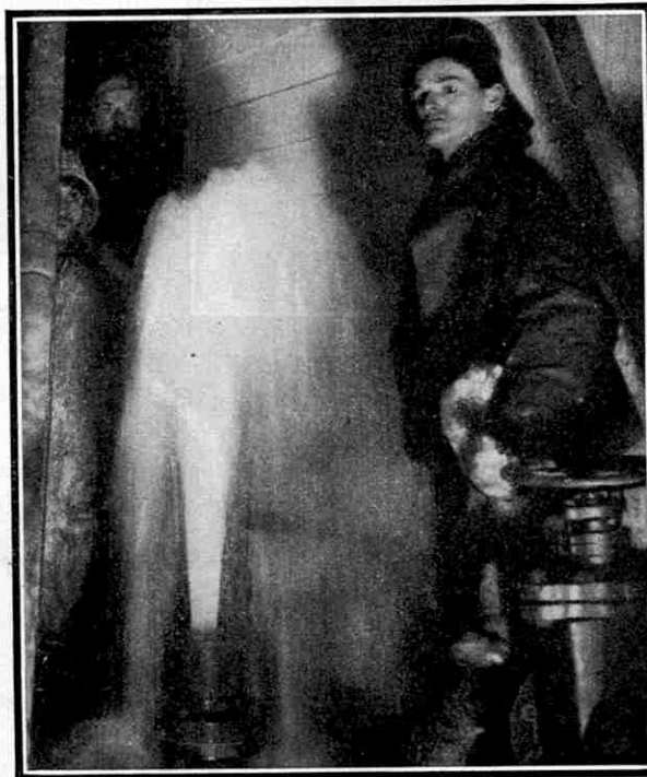
An artesian well overflowing. For the illustrations to this article we are indebted to Le Grand, Sutcliffe & Gell Ltd., London.
