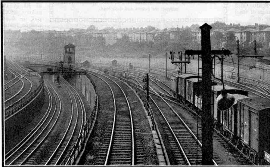
A view of some of the complicated junctions in the neighbourhood of Camden. Great use is made of flying and burrowing junctions to avoid the conflicting of different kinds of traffic.
