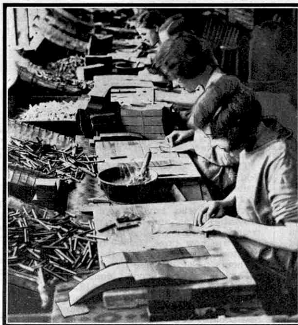
Rolling the cases for fireworks in the Standard Factory at Huddersfield.
