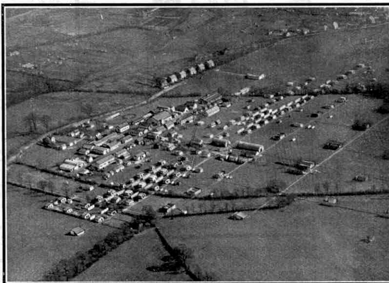
An aerial view of the Brock factory at Sutton. The metal screens separating individual workshops are clearly shown. For this photograph and the upper one on the next page we are indebted to C. T. Brock & Company Ltd.
