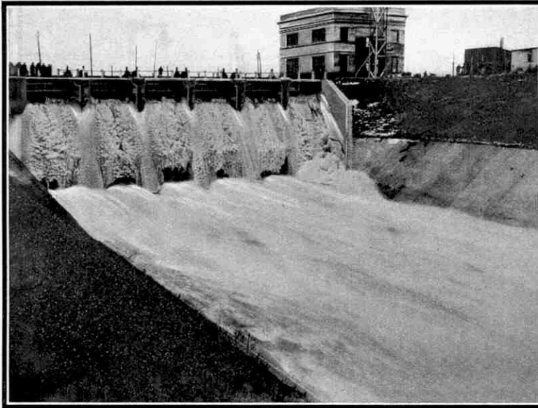
Testing the operating equipment of the weir that regulates the level of the water in Lock No. 1 of the Welland Ship Canal. It will be seen that this photograph was taken in wintry conditions.
