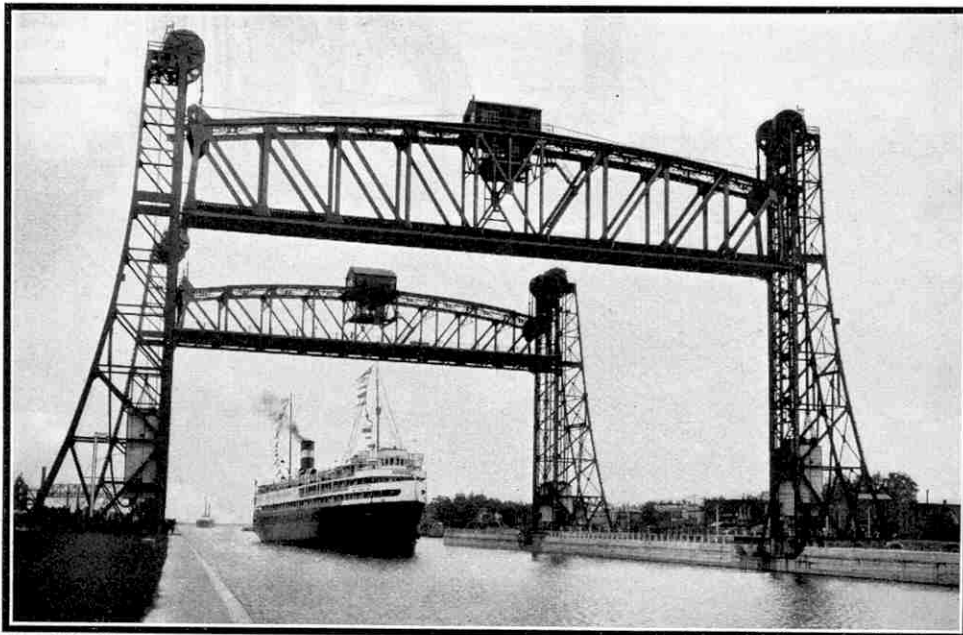
Two of the lift bridges of the Welland Ship Canal open to allow the passage of a large lake steamer entering the Canal from Lake Erie. There are 20 bridges across the Canal, and 10 of them are similar in type to those shown in our photograph. We are indebted to the courtesy of the Department of Railways and Canals, Canada, for the illustrations to this article.
