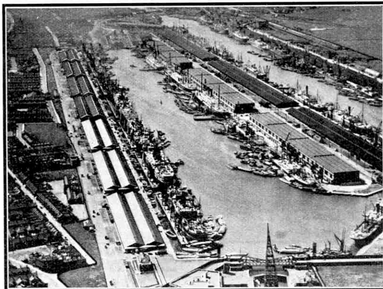
Looking down on the King George V and Royal Victoria and Albert Docks, which have a total water area of 246 acres and form the largest sheet of enclosed dock water in the world.
