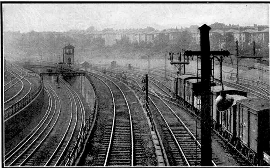
A view of some of the complicated junctions in the neighbourhood of Camden. Great use is made of flying and burrowing junctions to avoid the conflicting of different kinds of traffic.
