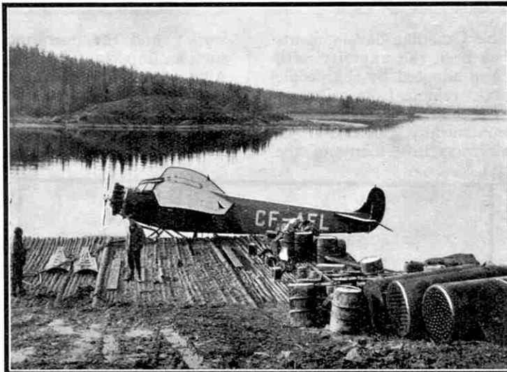
A Fokker Super-Universal seaplane used for carrying mining supplies to outlying Canadian territory. Skis are fitted to the machines during winter so that they can alight on the frozen lakes. An article dealing with the work of Canadian Airways Ltd., to whom we are indebted for the photographs on this page, appears on page 194.
