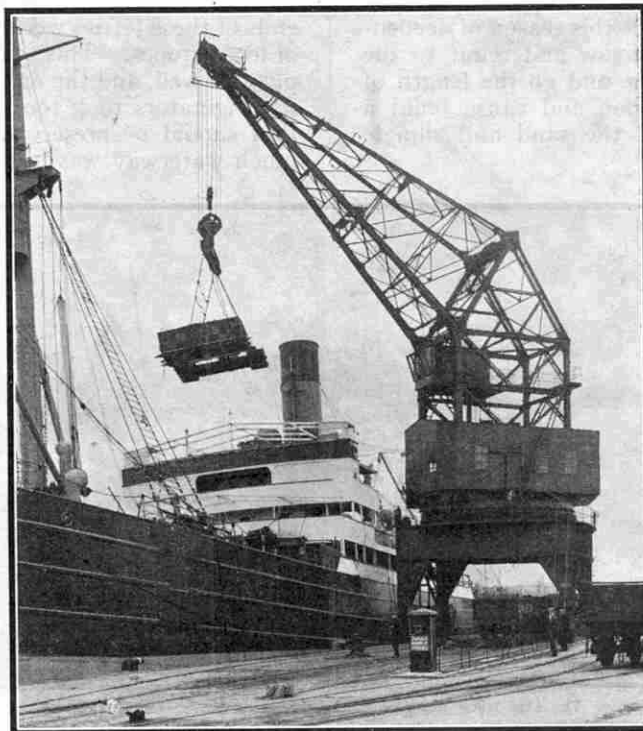
A 40-ton Electric Coaling Crane at work, Glasgow Harbour.
