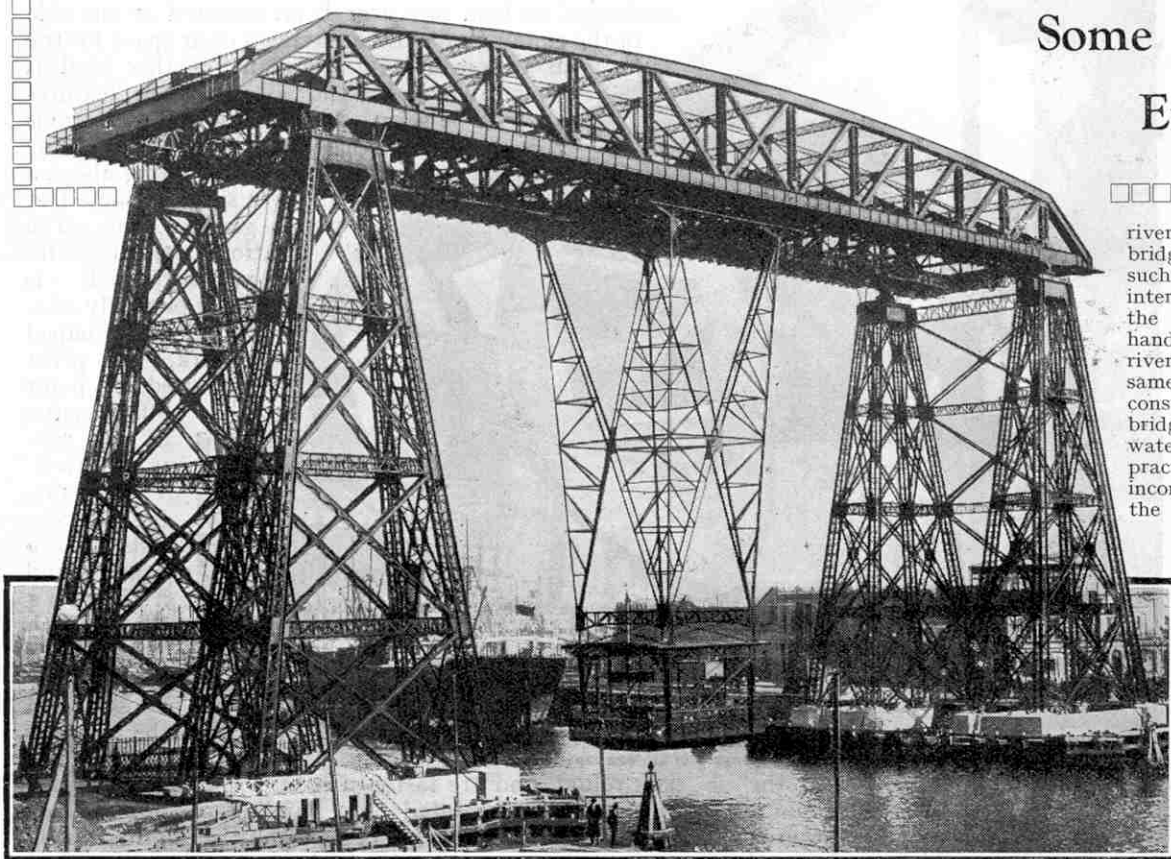
The Riachuelo Transporter Bridge, Buenos Aires, that crosses the River Riachuelo in a single span 854 ft. 3½ in. in length from the centres of the towers.
