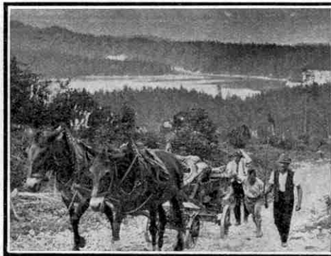
Portable compressors being conveyed in sections up a mountainside from the Eibsee.
