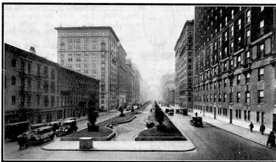
Photograph taken from the same point as the top illustration, after the electrification of the railroad, which runs beneath the Avenue. This shows the great improvement effected as a result of the covering in of the lines.
