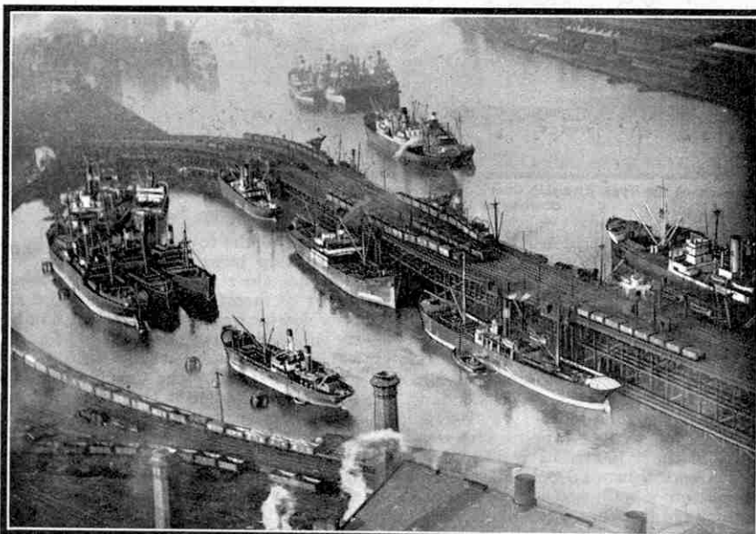
Looking down on Dunston coal staitths. Photograph by courtesy of the "Newcastle Chronicle."
