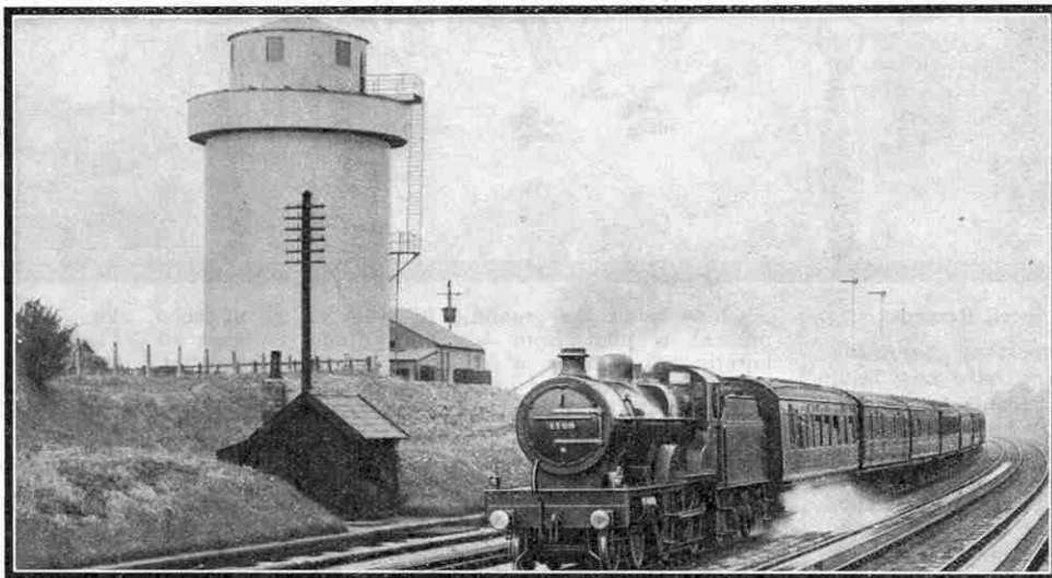
The softening plant and water troughs at Castlethorpe on the L.M.S.R. The plant operates on the L.H. Continuous-Automatic system perfected by the United Water Softeners Ltd., to whom we are indebted for this and the illustration on the previous page, and for information incorporated in this article.
