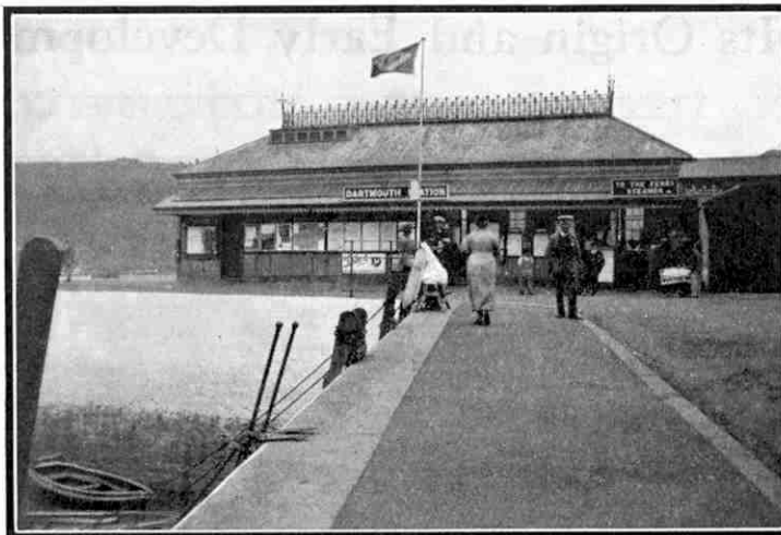
A railway station in which there are no rails! Photograph by R. Wood, Manchester.
