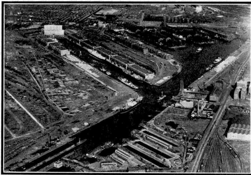
Aerial view of Manchester deep-water docks. Mode Wheel Locks can be seen at the left-hand bottom corner, and the dry docks are to the right. The illustrations on this and the opposite page are reproduced by courtesy of the Manchester Ship Canal Company.
