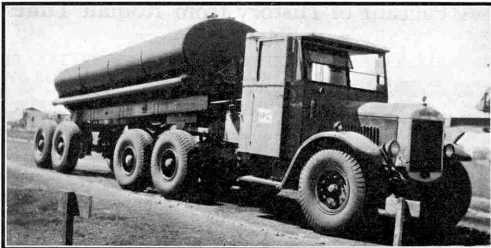
One of the nine Thornycroft 2,500-gall. tank lorries used in connection with the construction of the line. Photograph by courtesy of John I. Thornycroft and Co. Ltd.
