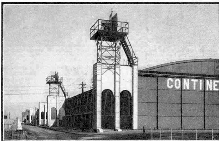
The large reflectors used for transmitting micro-rays, or very short wireless waves, from the aerodrome at Lympne to that at St. Inglevert, France. These reflectors are mounted on the roof of one of the hangars, and the aerials used in conjunction with them are only an inch in length.
