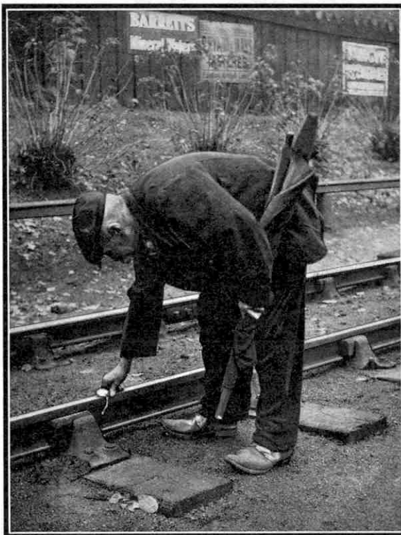
A fogman placing a detonator on the railhead, where it is secured by means of the soft metal clips, one of which is shown in the photograph. The illustrations to this article are by G. South, of Southport.
