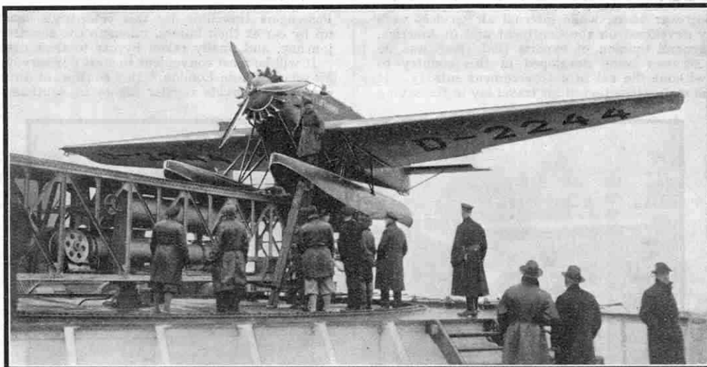
A Junkers seaplane on the catapult apparatus installed on the German liner "Bremen." By catapulting the aeroplane into the air while the vessel is still at sea, the delivery of urgent mails is considerably speeded up.
