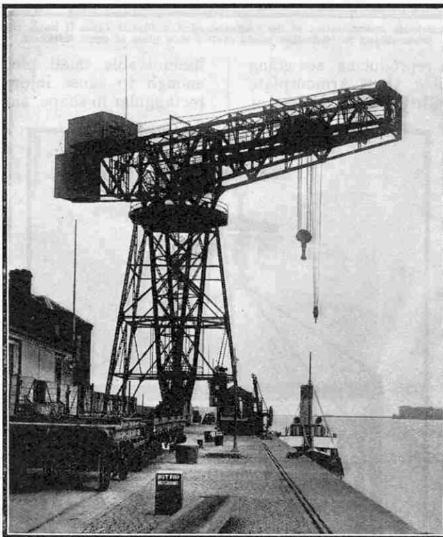
The 100-ton electric crane at North Wall Extension, Dublin. The illustrations in this article are reproduced by permission from "The Port of Dublin," published for the Dublin Port and Docks Board by Wilson Hartnell & Co., Dublin.
