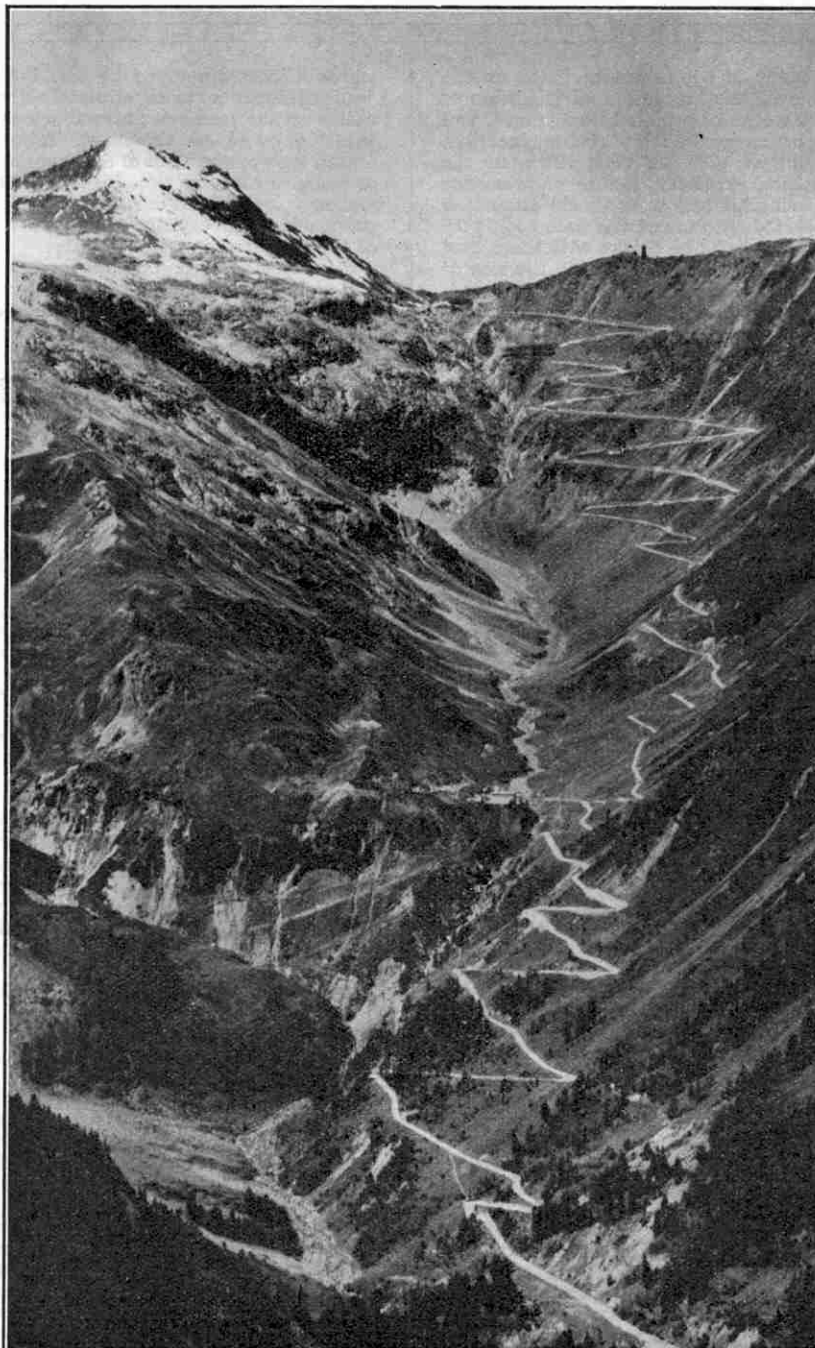
The wonderful motor road over the Stelvio Pass, in the Italian Alps. This road has 49 hairpin bends in its ascent of 12½ miles to a height of 9,050 ft. Photograph by courtesy of Frazer Nash Cars.
