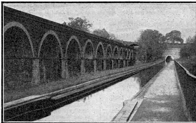
The upper photograph shows the Menai Suspension Bridge across the Menai Straits, probably the best known of Telford's works. It is 1,710 ft. long, and the road deck is 100 ft. above high water mark. The lower photograph shows the Ellesmere Canal, on the top of Chirk Aqueduct, and on the left is Chirk Viaduct.
