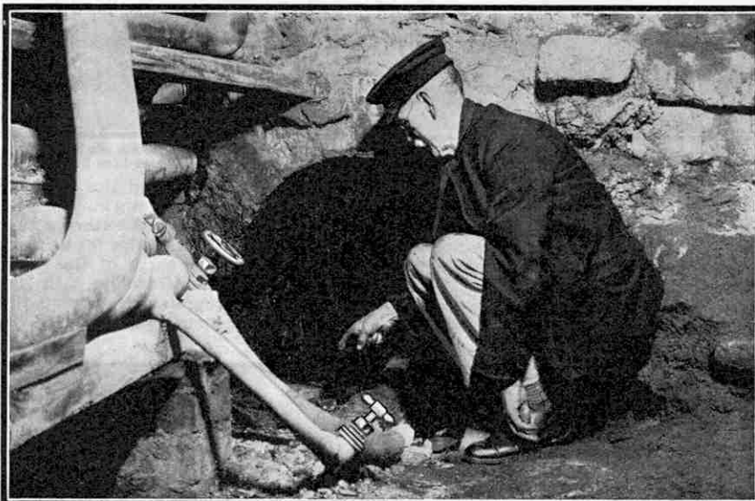
The subterranean passage through which pass pipes carrying 4,000 gallons of spa water daily to the Royal Mineral Water Hospital, Bath. Photograph by V. Chamberlain, Bath.
