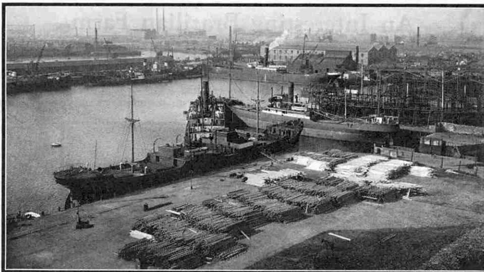
One end of the Alexandra Basin, which has a total water area of 60 acres and is deep enough to enable ships up to 32 ft. draught to lie afloat at all states of the tide.
