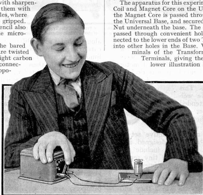
A magnetic surprise. A ring of aluminium is repelled by an electro-magnet actuated by alternating current.
