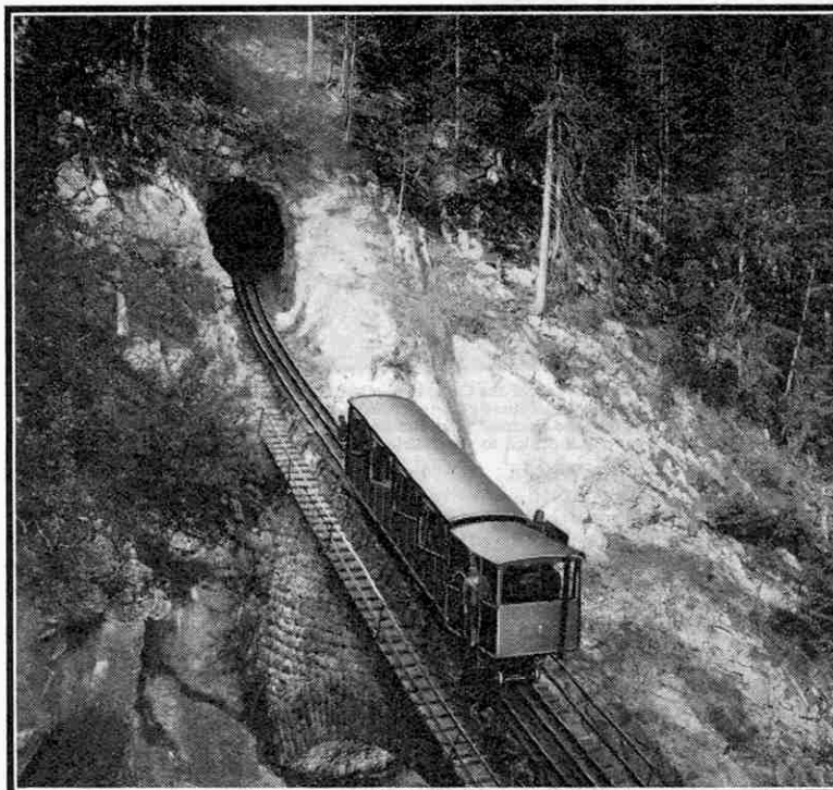
Emerging from a tunnel on to the Wolfort Viaduct on the Pilatus rack railway. The steam coach shown is of special construction in view of the severe gradients.
