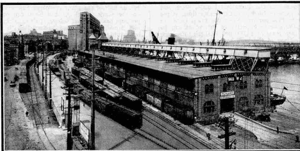
Typical two-storey transit shed with overhead conveyor-gallery.
