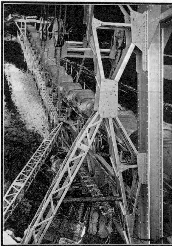
The boom of the machine. The empty buckets can be seen travelling outward, and above are the wire ropes from which the boom is suspended.
