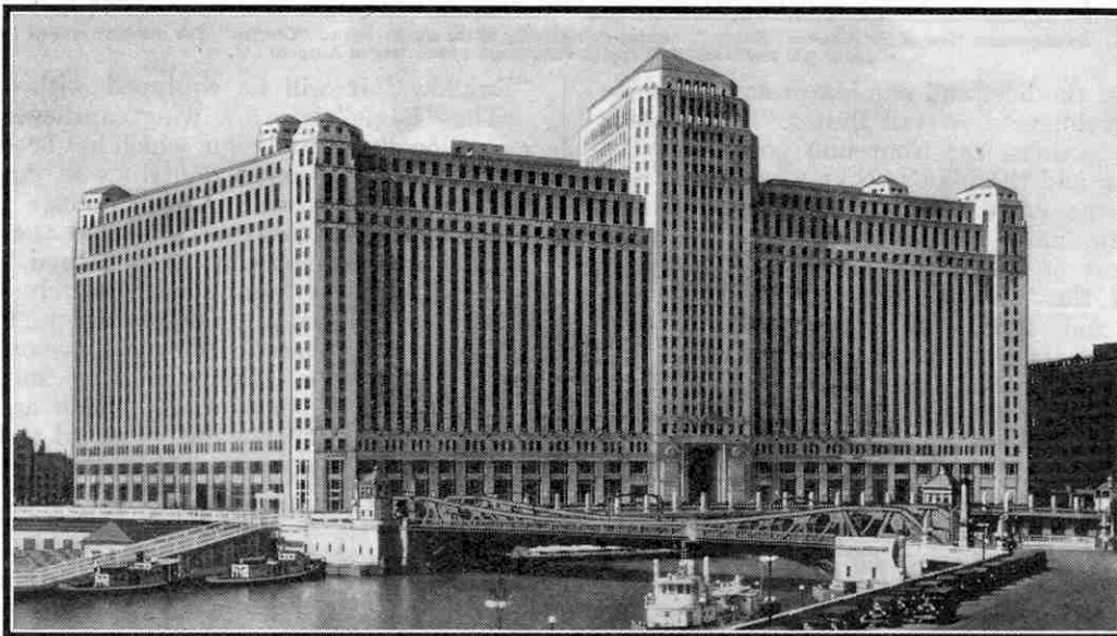
The river frontage of the Merchandise Mart, Chicago. The illustrations to this article are reproduced by courtesy of Messrs. Graham, Anderson, Probst and White, architects for the building.
