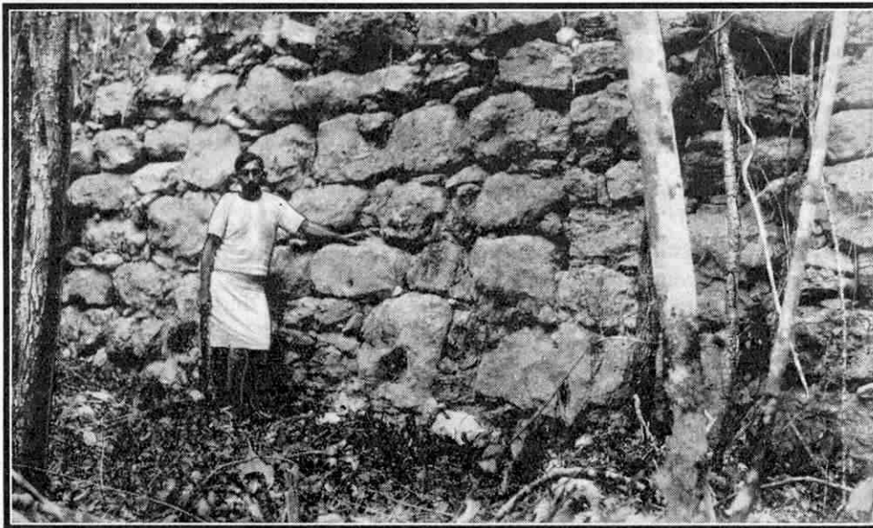
The Maya causeways were raised above the general ground level. This is a side view of one of them at its greatest height, 8 ft.
