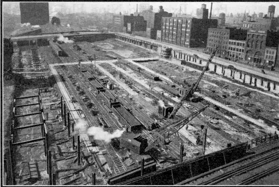
Preliminary work on the site of the Merchandise Mart, which is built on a foundation of 458 caissons sunk to a depth of 100 ft. below street level. The railway tracks now under the building can be seen in the background.
