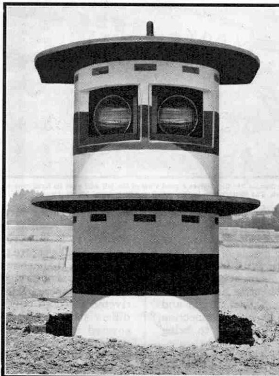
A rotating floodlight beacon that is a conspicuous feature of the lighting equipment at the National Air Port at Madrid, Spain. Photograph by courtesy of the International General Electric Company of New York.
