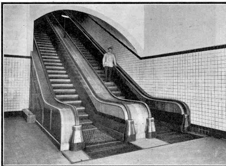
This illustration shows a set of escalators installed in the pedestrian tunnel.
