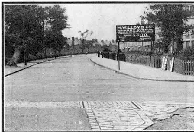
Part of the old tramway in modern surroundings. In the foreground are two rails still in place although almost enclosed by stone sets.
