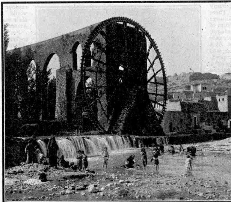
The largest of the four waterwheels at Hama. This is 75 ft. in diameter and is probably the largest water-raising wheel in existence.
