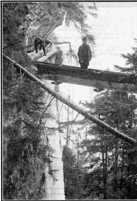
A precarious position on the footpath by the side of a "bisse" or waterway, on a Swiss Mountain. A bisse is a narrow channel in which water is brought from glaciers to the valleys below, and our photograph shows how one of these channels crosses a deep chasm.
