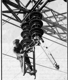
A structural worker making adjustments on the Boulder Dam-Los Angeles power line.
