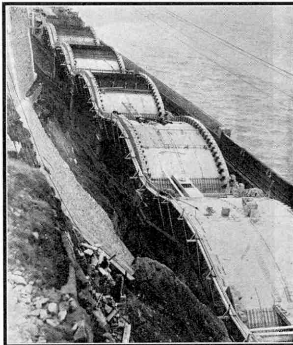
The viaduct during construction, showing steel plating in position.
