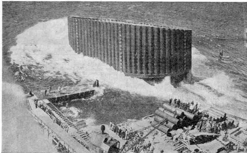
One of the specially-built caissons being launched from the slipway.
