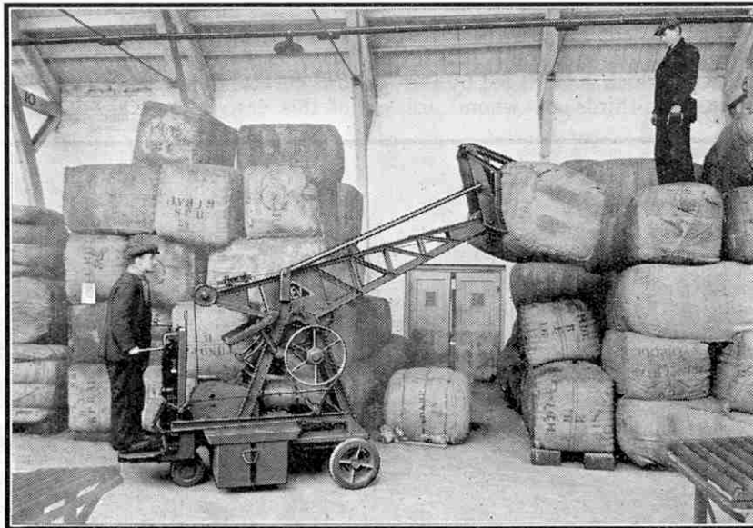
One of the Bale Stacking Trucks in use at Frizinghall, L.M.S.R., stacking bales of wool. Illustration by courtesy of Wingrove and Rogers Ltd. of Liverpool, the makers of the truck.
