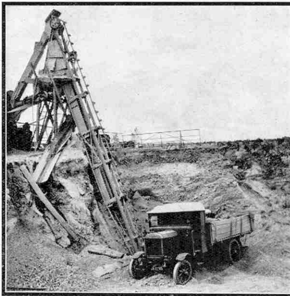
A bucket elevator feeding gravel into a washing and grading plant.
