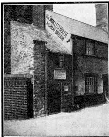
This house at Conway is claimed to be the smallest in Great Britain. Photograph by J. Thomas, Glasgow.
