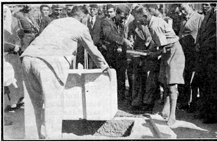
The laying of the foundation stone of the Kut Barrage by the King of Iraq, who is seen lifting mortar with a trowel. Photograph by J. G. Abbood, Baghdad.
