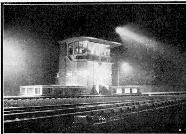
A striking night photograph of the control tower. This shows the adjacent floodlighting unit that is used for "spotting" the progress of the wagons.
