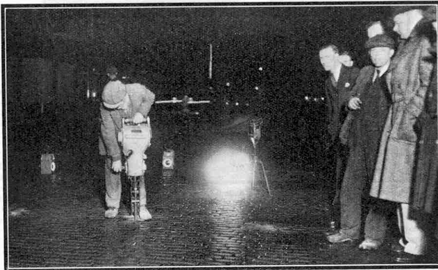
The Warsop Road-Breaker in use. This tool is self-contained, the digging spike being operated by a two-stroke petrol engine. The illustrations on this page are by courtesy of George Cohen, Sons and Co. Ltd.
